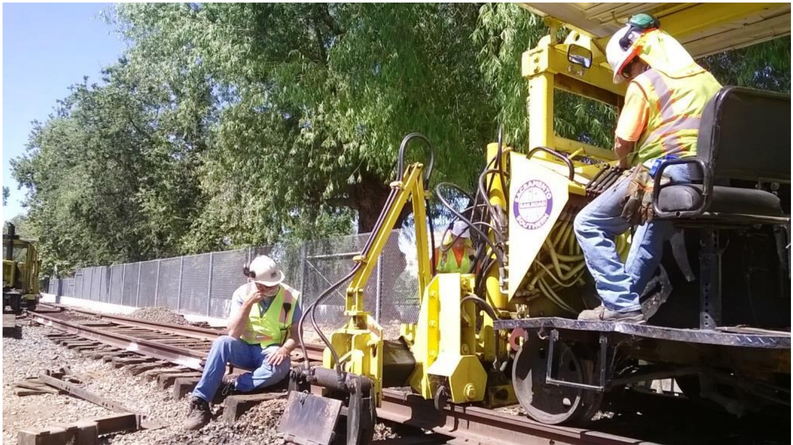
Alan contemplates the placement of the ties as Joe draws them under the rails
