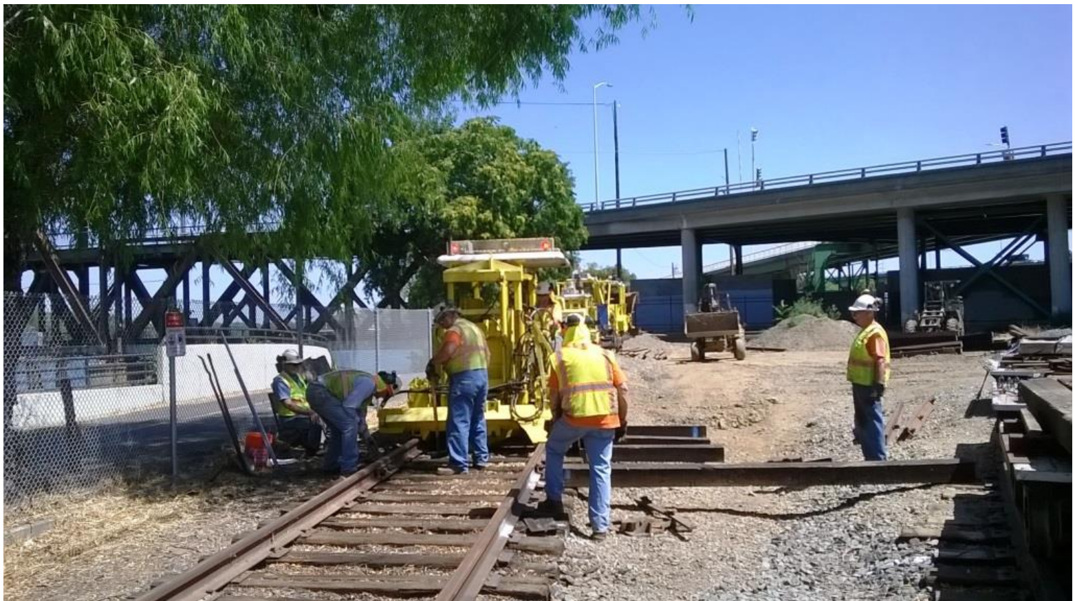
The Team works with the Jackson 125 as it pulls-in the extra-long ties
