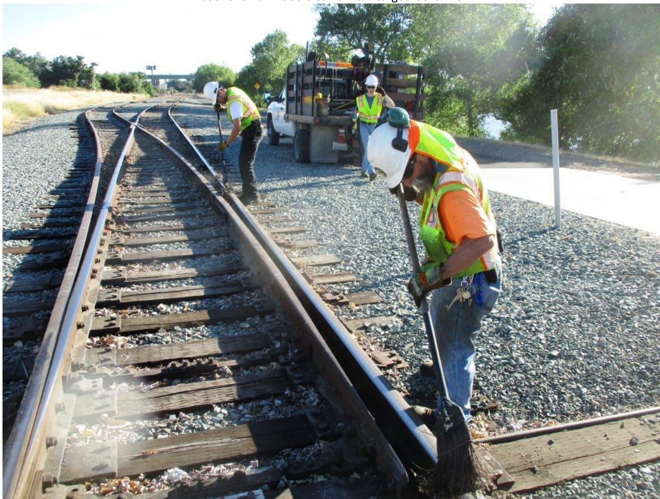
Kyle and Joe clean debris from between the switch-point and stock rail
