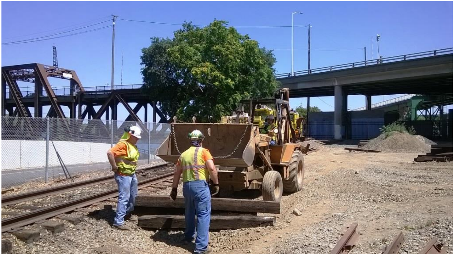
Using the timber tong attachment, Ed moves these heavy ties with Bill and Mike F.'s help
