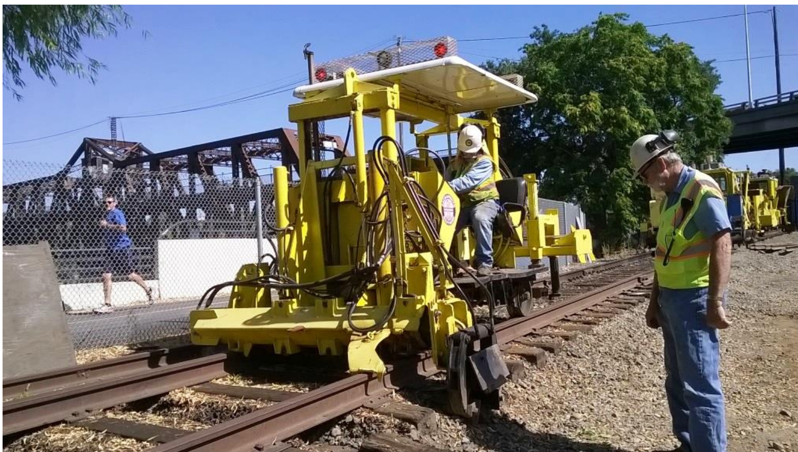
Alan keeps a keen eye on Joe and the 125 as ties are pulled
