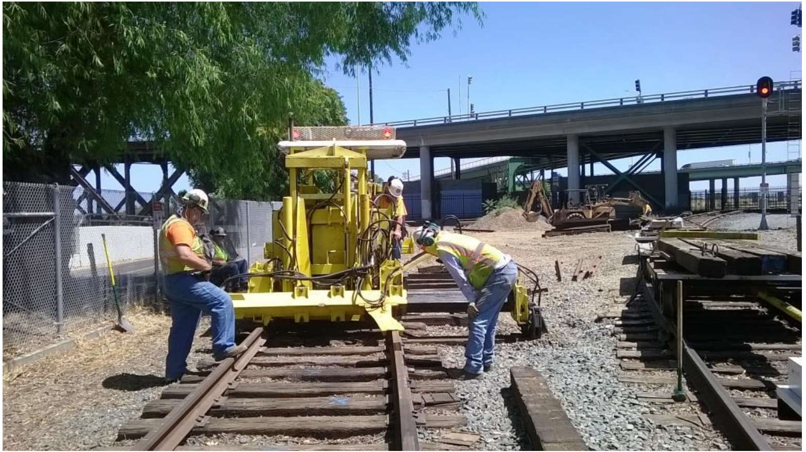
Mike F. and Steve watch to make sure the new tie gets spaced properly
